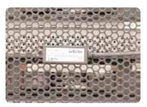
An example of a temperature sensor mounted at the cold air inlet of a server rack. Sensor is connected to an intelligent PDU (not shown).
